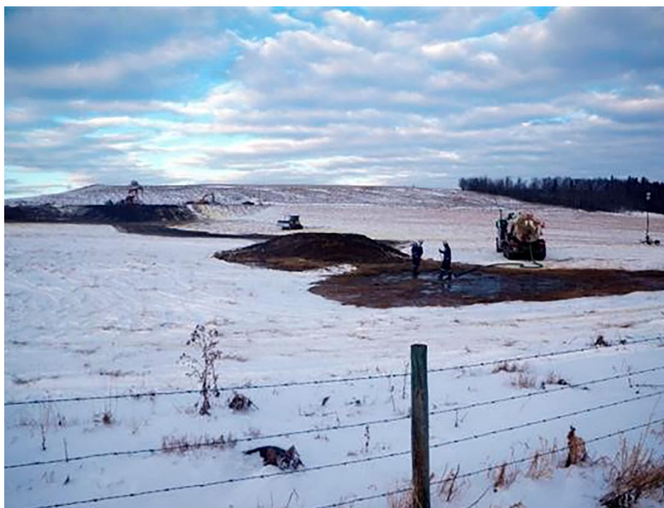
Figure 16 - Inter-wellbore communication event, Innisfail, Alberta, Canada, January 2012 (photo from Calgary Herald, January 17, 2012). Hydraulic fracturing fluids injected at one well were discharged under high pressure from another well to land surface.
