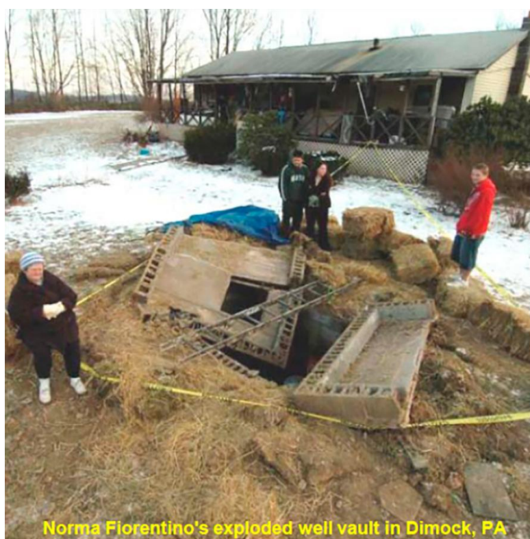
Figure 19 - An exploded water-well vault near drilling operations in the Marcellus Shale gas play, Dimmock, Pennsylvania, January 1, 2009 (adapted from Soeder, 2012).
