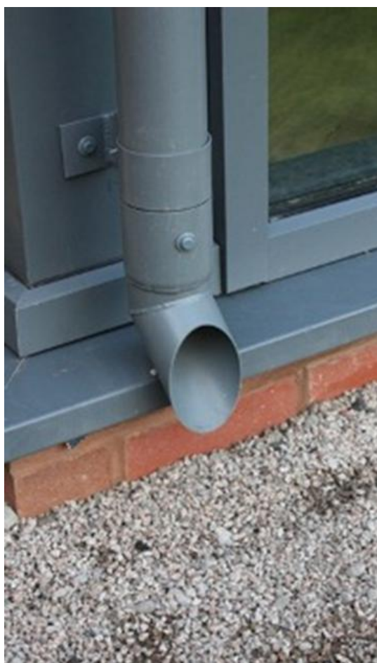
Figure 13 - Downspout disconnection programs in Toronto, Canada, help resolve stormwater management problems but are not quantitatively assessed and, in the absence of water level monitoring, may easily overload the aquifer system and cause flooding of basements, tunnels, and electrical utilities. In Toronto, Canada, landslides along the Scarborough Bluffs are primarily facilitated by the discharge of groundwater (also Section 3.2, Aquifer Outflow (Discharge) ) (photography by Ken Howard).
