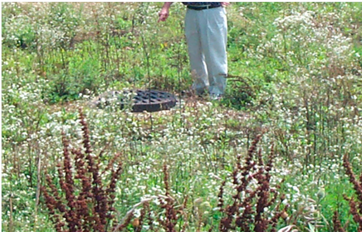
Figure 87 - Recharge basin for the infiltration of stormwater on Long Island, New York, USA. The basin requires very little maintenance since the roots of vegetation maintain sufficient soil permeability (photography by Ken Howard).
