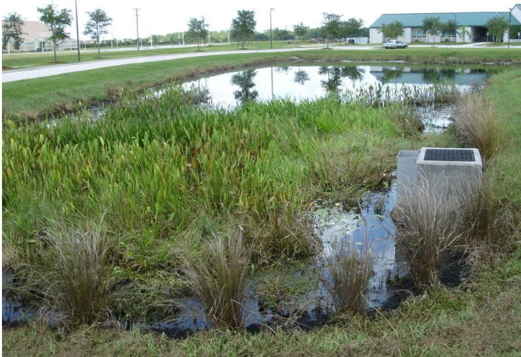
Figure 46 - Wet stormwater detention pond: an earthen pond with a permanent pool and temporary storage for attenuating stormwater flows (photography by the Georgia Department of Transportation, USA).
