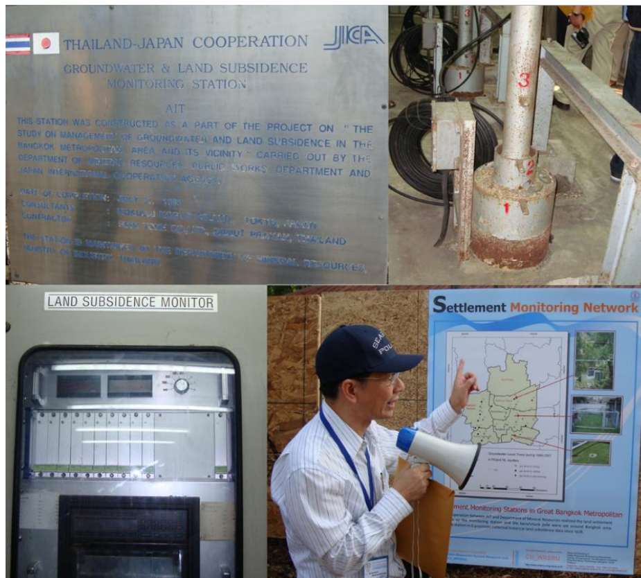
Figure 76 - In Thailand, the task of combating land subsidence has relied heavily on data provided by the country's settlement monitoring network (photography by Ken Howard).
