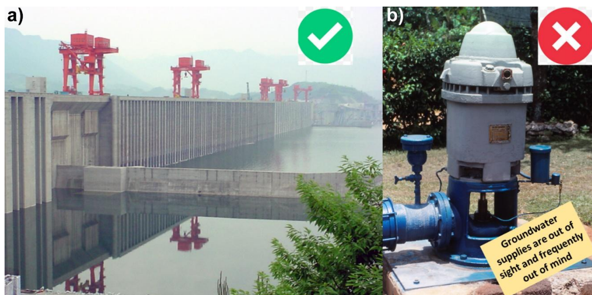
Figure 121 - Global investment in water has always favored spectacular, expensive, but easily monitored surface water schemes such as dams and pipelines over low public-profile wellfield developments involving “invisible” groundwater. Figure a) shows the Three Gorges Dam (China), and b) shows a municipal well near Kingston, Jamaica (Photography by Ken Howard).
