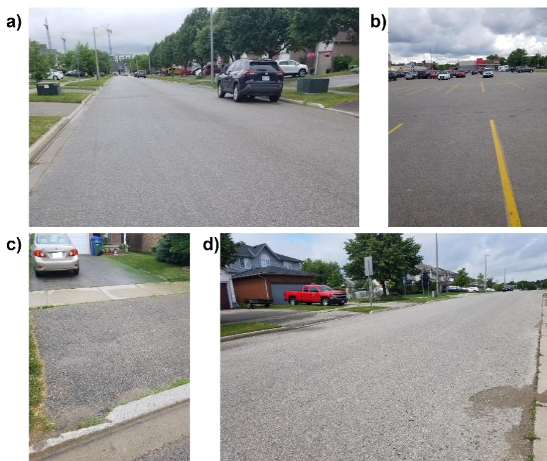
Figure 9 - Impermeable cover in an urbanized watershed includes paved a) roadways, sealed roads, b) parking lots, c) and d) sidewalks, pedestrian pathways, and roofs. In practice, it may also include sports fields and parks where underground drains have been installed to intercept any water that is in excess of basic evapotranspiration requirements (photography by Jamie Bain).
