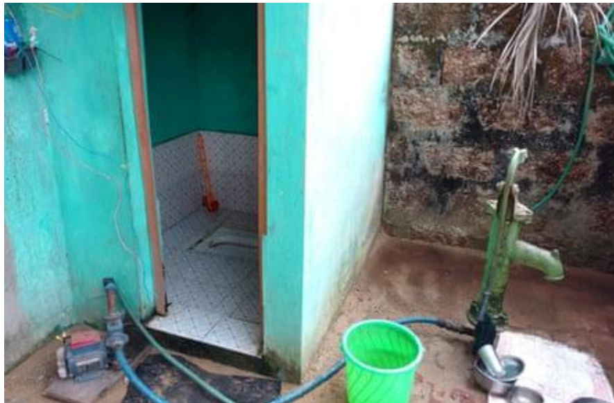
Figure 95 - A study in northern India found evidence of fecal contamination in 18 percent of the water sources; 91 percent of the contaminated water sources were situated within 10 m of a recently installed toilet (Pulla, 2016).
