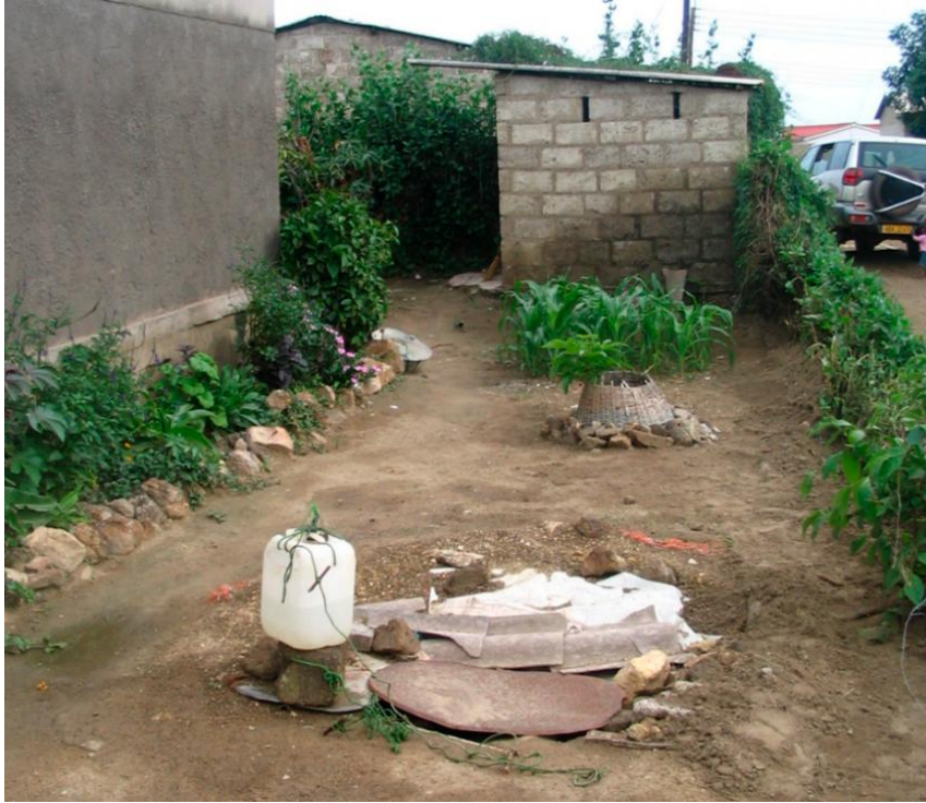
Figure 94 - Example of groundwater pollution in Lusaka, Zambia, where the pit latrine in the background is contaminating the shallow well in the foreground with pathogens and nitrate (photography by Kennedy Mayumbelo).
