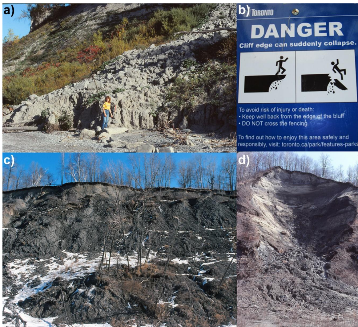
Figure 20 - a) Regular landslides along the Scarborough Bluffs, Toronto, Canada, are primarily facilitated by the discharge of groundwater (Eyles & Howard, 1988), despite statements by the local conservation authority that landslides are mostly related to water levels in adjacent Lake Ontario. Locally, groundwater discharge is enhanced by downspout disconnection programs that redirect potential stormwater flows to the subsurface (Figure 14). b) In some locales, the resulting land instability limits use of lands that would benefit the community (photography by Ken Howard).
