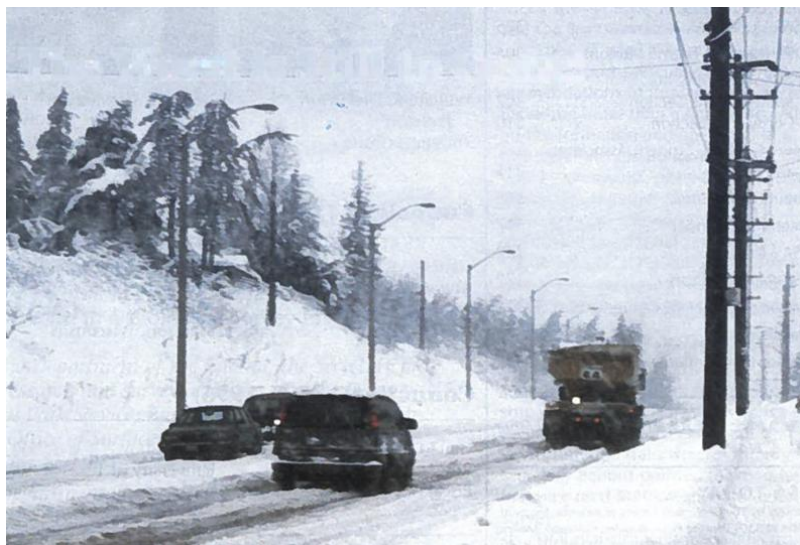
Figure 42 - In snow belt regions of the world, application of road de-icing salts is the only cost-effective means of maintaining the flow of traffic on roads and highways (photography by Ken Howard).
