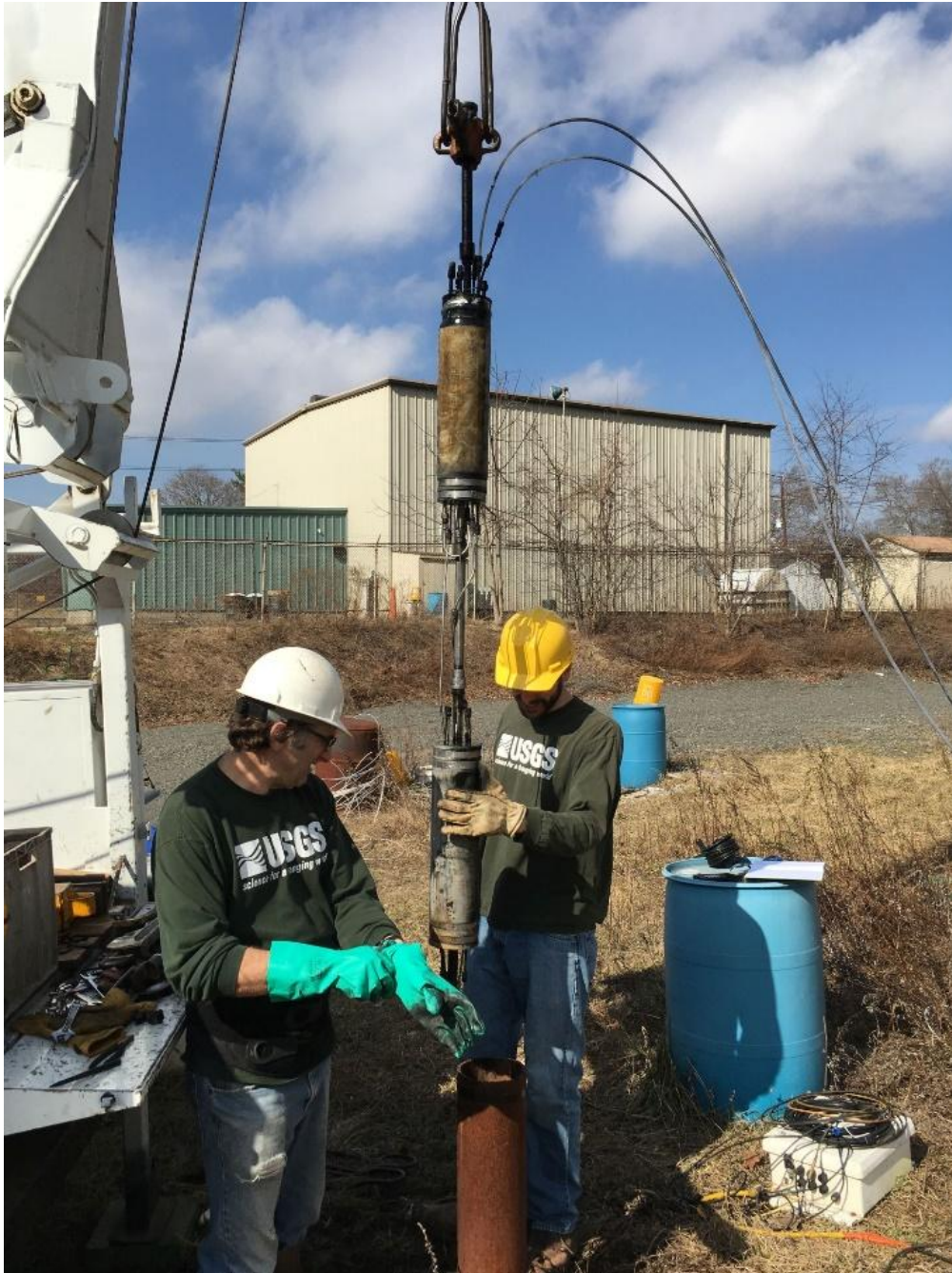
This photograph shows the installation of two packers used to isolate a section of open borehole ( http://www.usgs.gov/media/images/photograph-usgs-hydrologists-and-packers-well-testing ).
