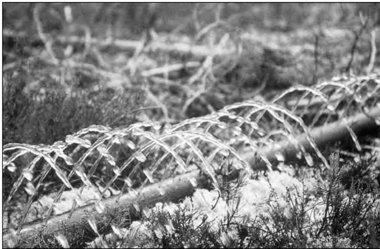
Figure 1.12 Low-pressure perforated pipe for aquifer recharge in Finland
