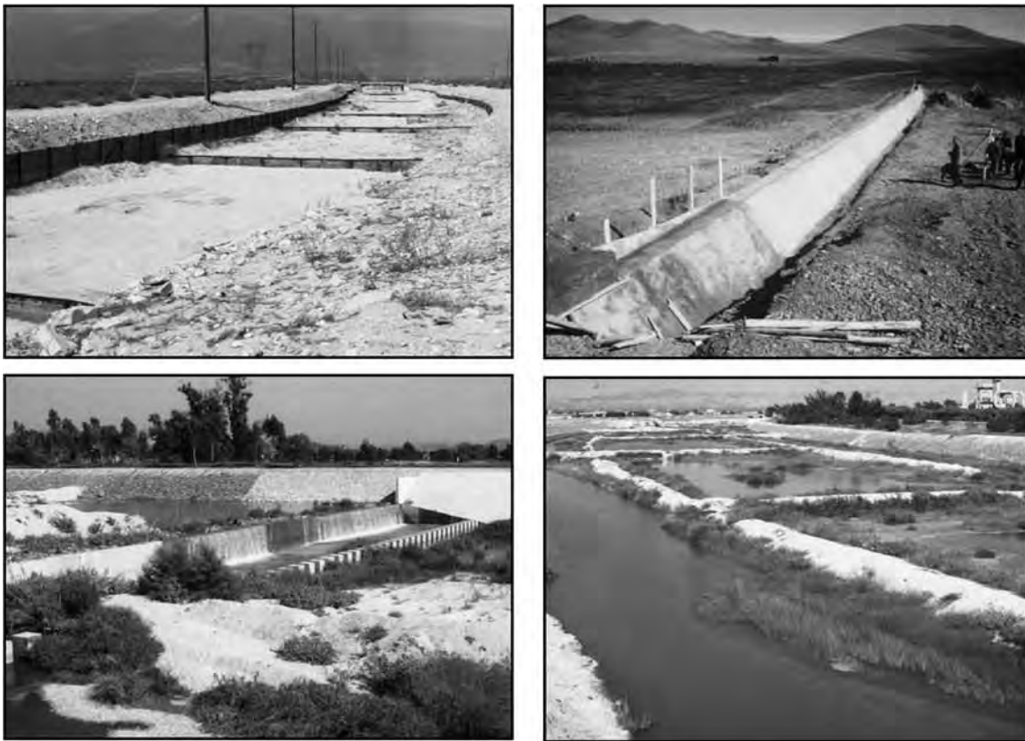
Figure 1.6 Photos of in-channel infiltration systems with low weirs in narrow, steep channel (top left); a 2 m high concrete dam in a wide Moroccan wadi (top right); a low dam in a more gently sloping channel (bottom left); and T-levees in wide, flat channels (bottom right)
