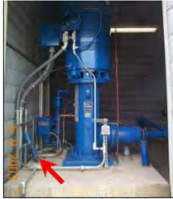
(a) Install extra water level tubes
