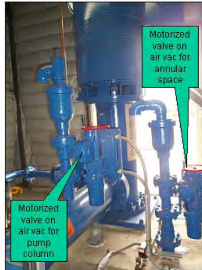
(c) Use MOVs to minimize air entrainment
