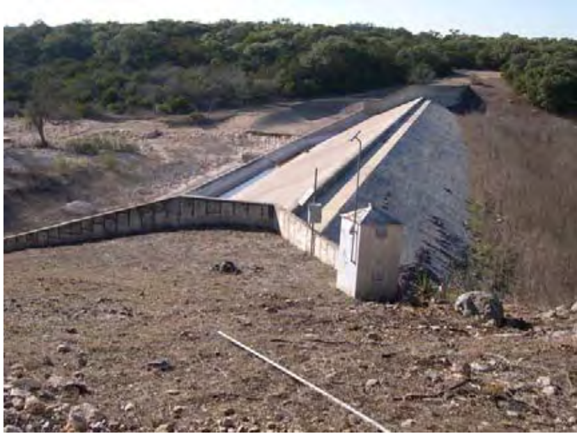
San Geronimo Creek Recharge Dam (February 2006)
