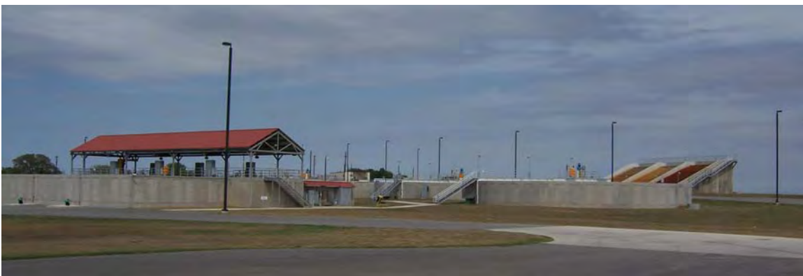
Figure 1: Water Treatment Plant (Morris, 2006)
