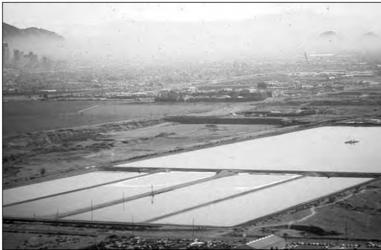
Figure 1.18 Polishing pond and four infiltration basins of 10 acres each for secondary sewage effluent in Phoenix, Arizona
