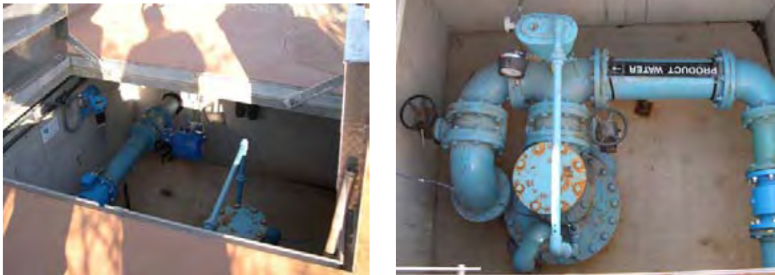
Figure 4: Standard Recharge Wellhead Configuration (Pugh, 2006)
