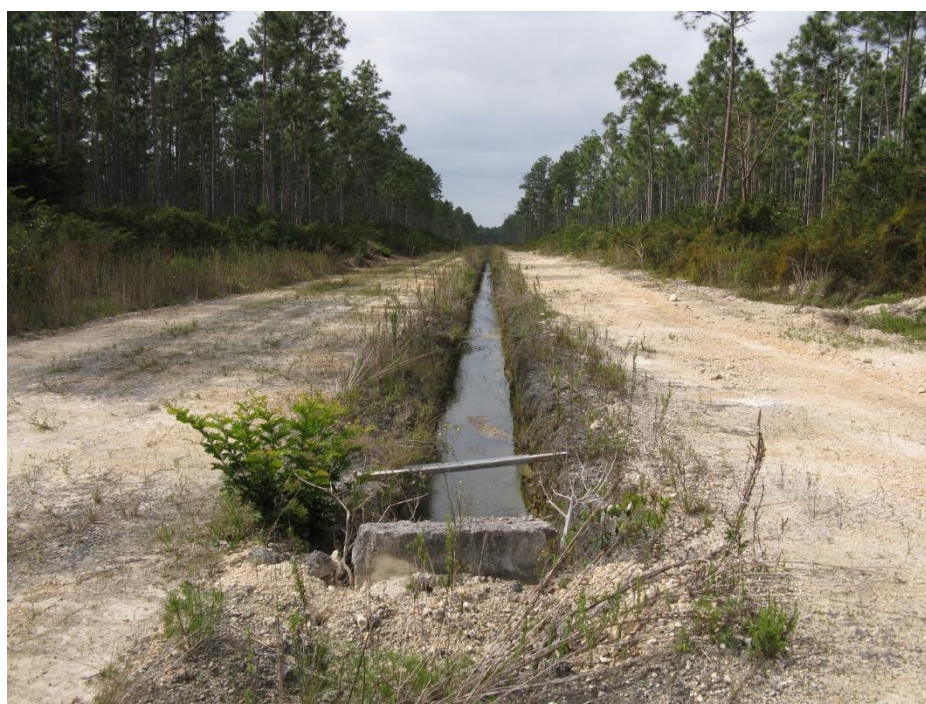
Figure 34 - Trench well on Andros Island, the Bahamas. The trench extends to a depth just below the water table and skims water from the freshwater lens on the island.
