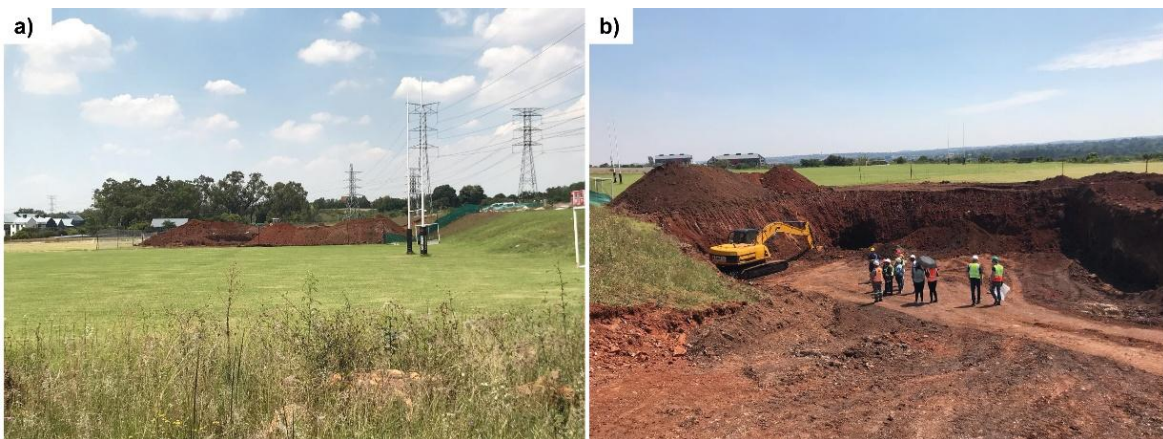
Figure 59 - Rehabilitation of a sinkhole in Pretoria: a) removal of collapsed overburden and b) excavated sinkhole showing maximum development space (photographs by van Rooy).
