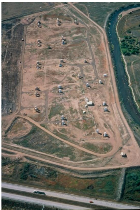
Figure Box 2-4 – DNAPL recovery Modules 1 (right) and 2 (left) at a former wood treating facility.
