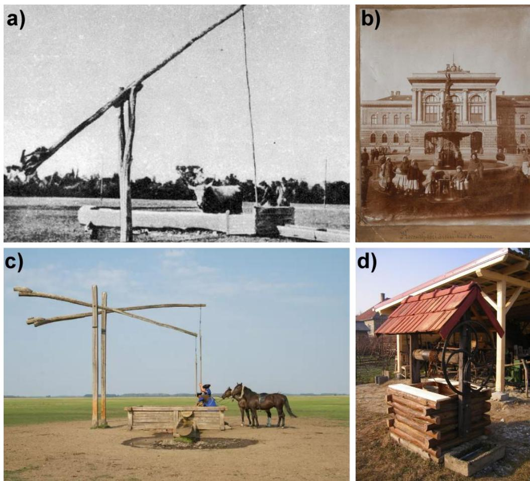
**Figure 5** - a) Draw (or sweep pole) well, late 1800s. b) Artesian well drilled in 1886 to a depth of 312 m in Szentes, Hungary. c) Modern day sweep pole well. d) Cable-wheel well (Bulgarian type). Photo credits:
