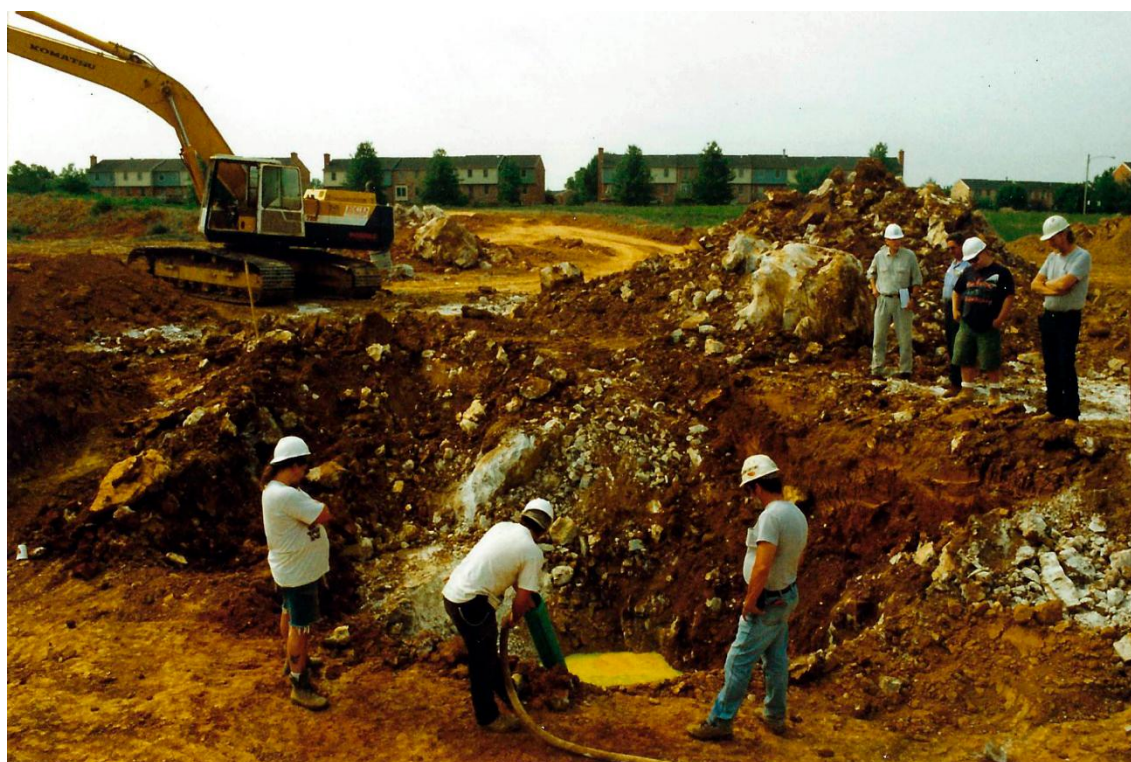
Figure Box 7-1 - Dye and flush water introduction at the re-excavated site of the pipeline rupture. The introduction of dye was followed by 8,100 gallons (30,800 L) of potable water delivered through a hose from a fire hydrant.
