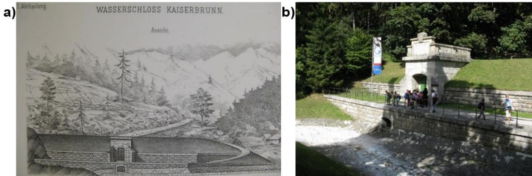
**Figure Box 21-1** - Vienna's engineering masterpiece. a) Original drawing of the Kaiserbrunn intake (courtesy of the Kaiserbrunn Museum, Vienna). b) Entrance to the spring intake today. Below the entrance gate is an evacuation channel for peak flows (photograph by Z. Stevanović).
