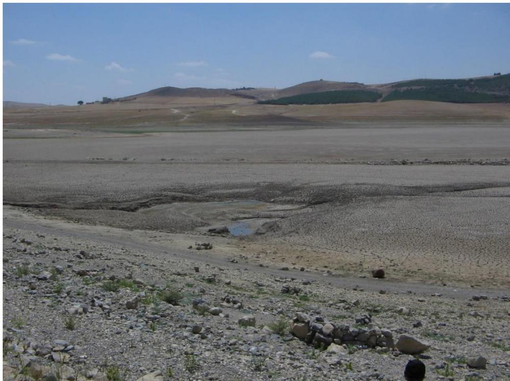
**Photograph Album 73** - An empty reservoir at Hammam Grouz in the karst of northern Algeria. Following remedial measures to reduce water losses, the reservoir operated successfully for about 20 years until several new swallow holes formed, completely draining the reservoir (photograph by Z. Stevanović).
