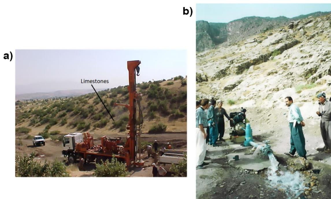
**Figure 57** - Drill operations: a) drilling limestone in the foothill zone, and b) pumping of the completed well used for irrigation of orchards in the Shaqlawa Plain, northern Iraq (photographs by Z. Stevanović).
