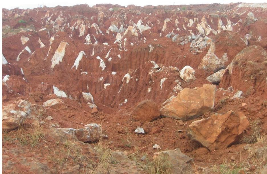
**Photograph Album 81** - As part of the development of the Kunming Changshui International Airport (Yunnan, China), which opened in 2012, soil and 'stone teeth' were removed from 23 km<sup>2</sup> of karst (photograph by N. Ravbar).
