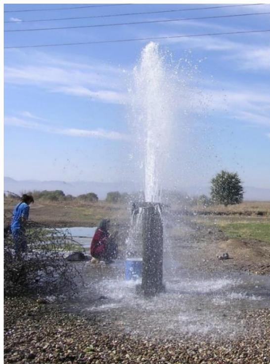
**Figure 82** - One of the *humanitarian* wells drilled during a drought in a confined karst aquifer near Said Sadiq (Iraq), with a dual purpose-potable water supply and irrigation (photograph courtesy of S. Ali, 2007).
