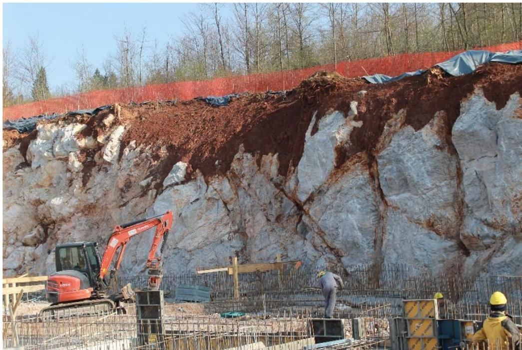
**Figure 75** - During construction, the protective layer of the aquifer is usually removed, increasing its vulnerability (photograph by N. Ravbar).
