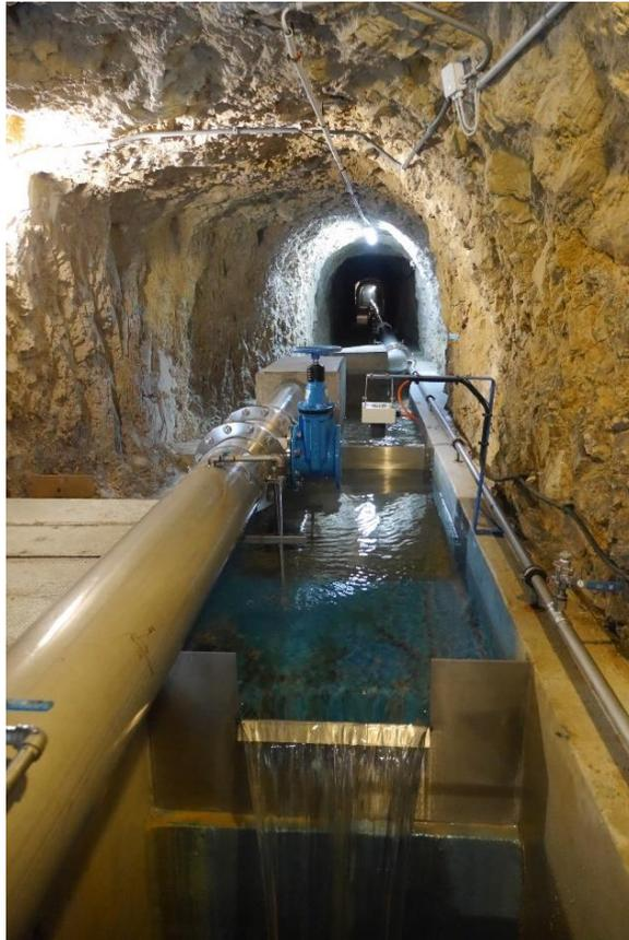
**Figure 56** - Karst water drainage gallery in the Areuse gorges for the drinking water supply for the city of La-Chaux-de-Fonds in the Swiss Jura Mountains (photograph by N. Goldscheider).
