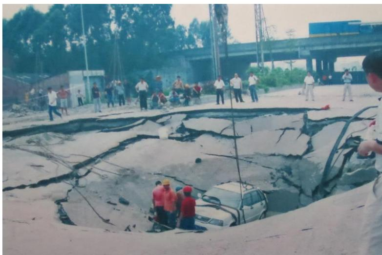
**Figure 81** - Dropout doline (sinkhole) that formed beneath a highway in Guilin, China (photograph courtesy of the Geological Museum of the IRCK, Guilin).
