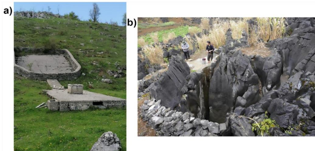
**Figure Box 20-1** - Water supply in high karstic mountain regions: a) rainwater collector in high mountains of the Piva River basin, Montenegro (photograph by Z. Stevanović); and b) water storage in an epikarst structure, Vietnam (photograph by N. Goldscheider).
