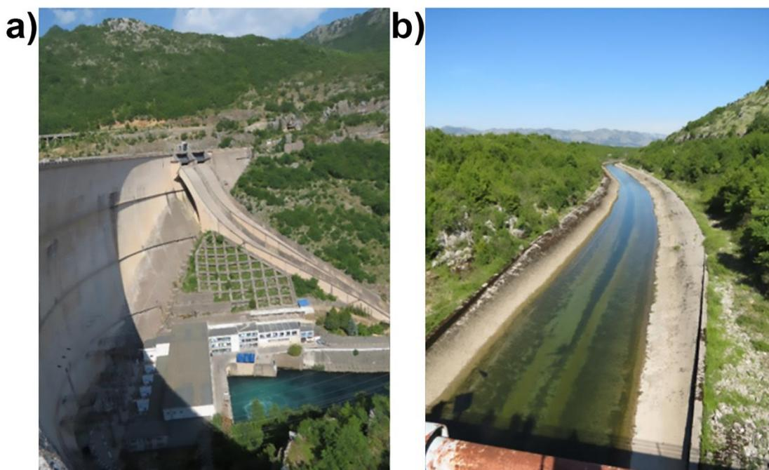
**Figure Box 27-1** - A successful large dam project in karst. a) Massive concrete arch dam Grančarevo and b) downstream channelled Trebišnjica River in the karstic Popovo polje, eastern Herzegovina (photographs by Z. Stevanović).
