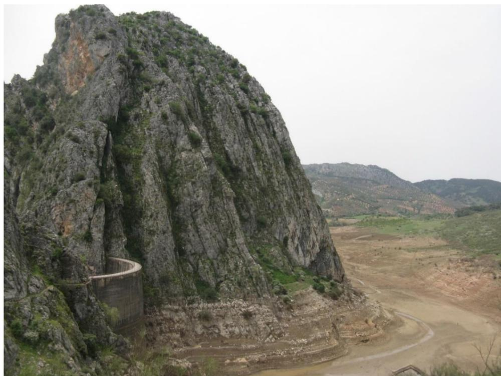
**Photograph Album 74** - The Montejaque dam in Andalucía, southern Spain, is a good example of the consequence of failing to understand karst hydrogeology. Built in the 1930s, the gravity arch dam is 84 m high and has an 84 m crest length. The reservoir has never completely filled with water due to the very permeable karstified rocks around the dam site and consequent water losses (photograph by Z. Stevanović).
