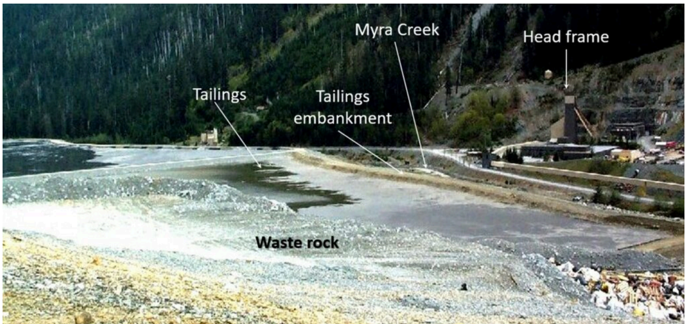
Figure 8.2.3 The Tailings Pond at the Myra Falls Mine on Vancouver Island. The dry rock in the foreground is waste rock. The structure in the background on the right is the head-frame for the mine shaft. Myra Creek flows between the tailings pond and the head frame, and the tailings embankment has been constructed to keep the tailings out of the creek.
