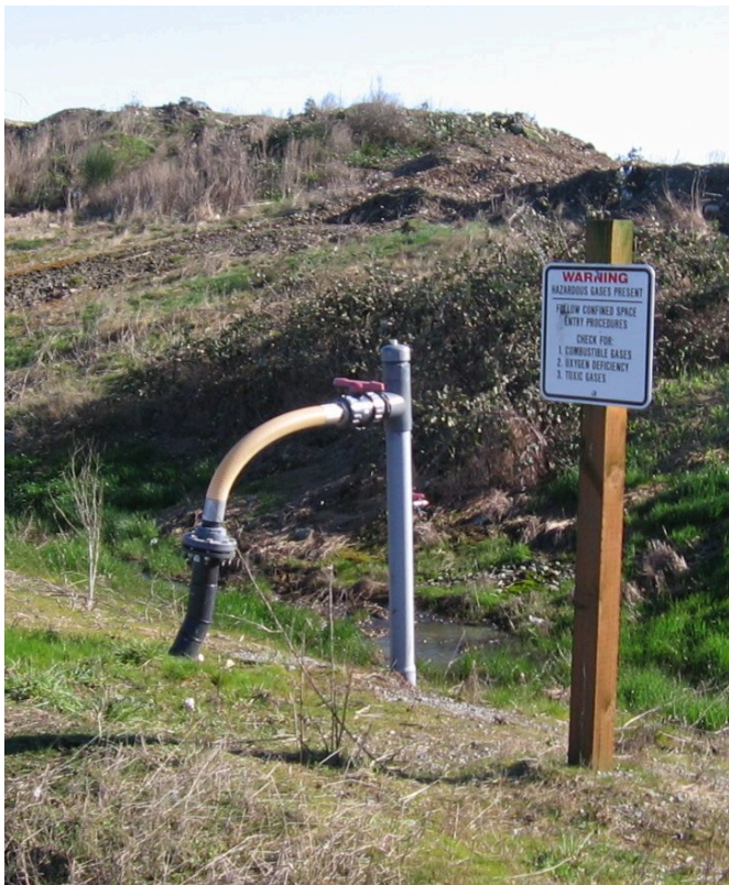
Figure 14.2.4 A Landfill Gas Wellhead. The vertical grey pipe penetrates the cover membrane and extends down into the waste. The flexible orange pipe connects to the gas collection system.
