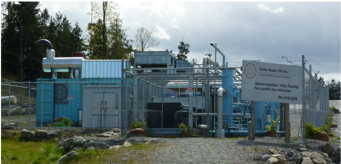
Figure 14.4.1 A Landfill-Gas to Electricity Plant at the Landfill Near to Nanaimo, BC
