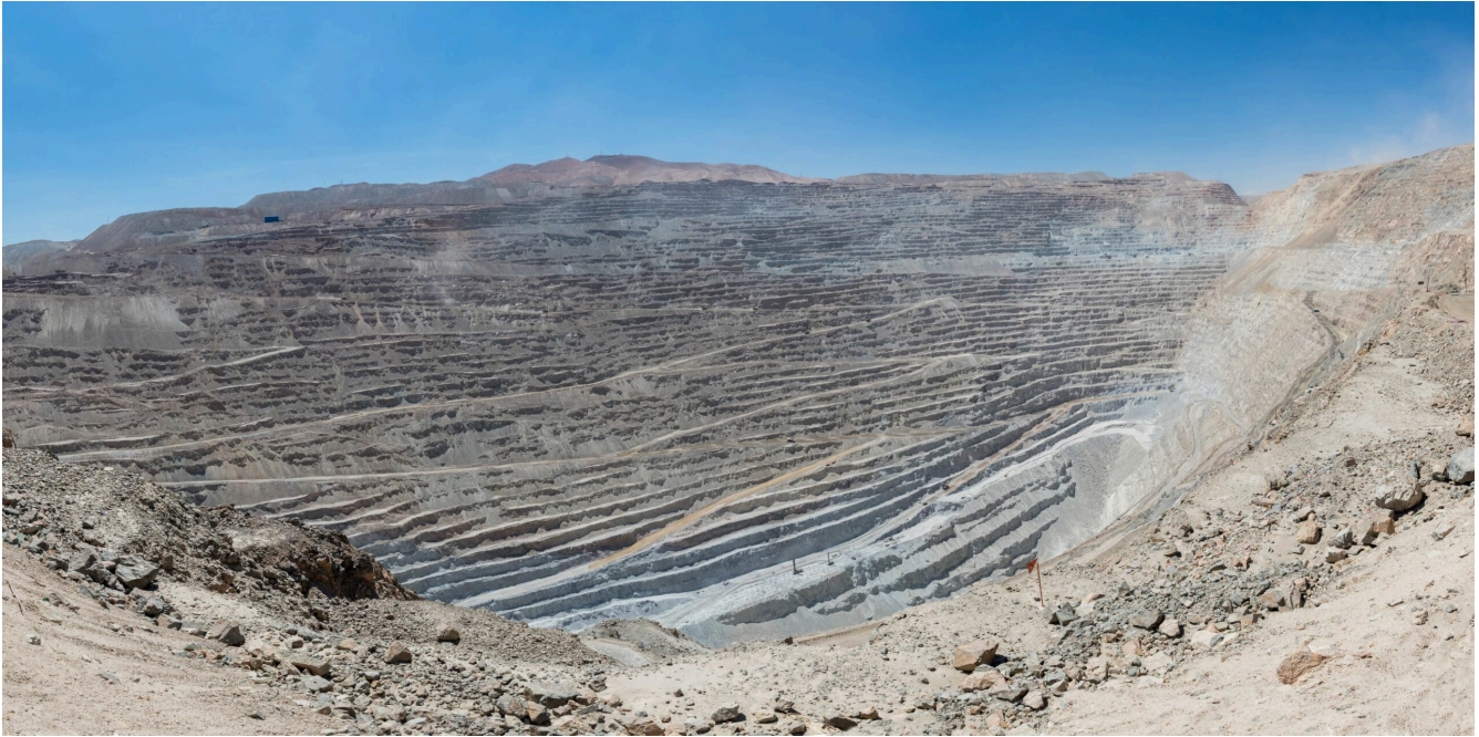
Figure 8.15 The Chuquibambilla Open Pit Copper Mine in Northern Chile. The pit is 4.3 km long, 2.7 km wide and 1.1 km deep. Mining currently takes place underground, below the bottom of the pit.
