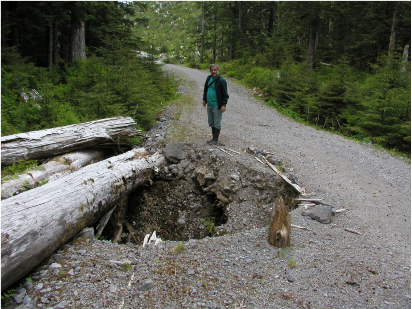
Figure 12.6.5 Redirection of Water Drainage on Karst Leading to Subsidence and Collapse of Road Fill Material, Southeast Alaska
