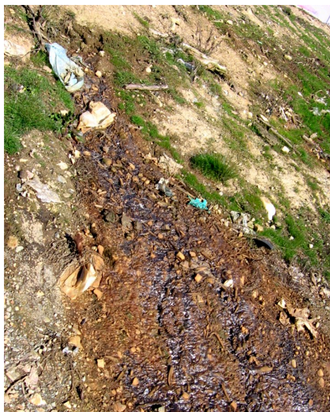
Figure 14.3.1 A Leachate Leak on the Flank of a Landfill at Nanaimo, Canada, Photo shows the formation of iron oxide minerals resulting from oxygenation of the leaking water.
