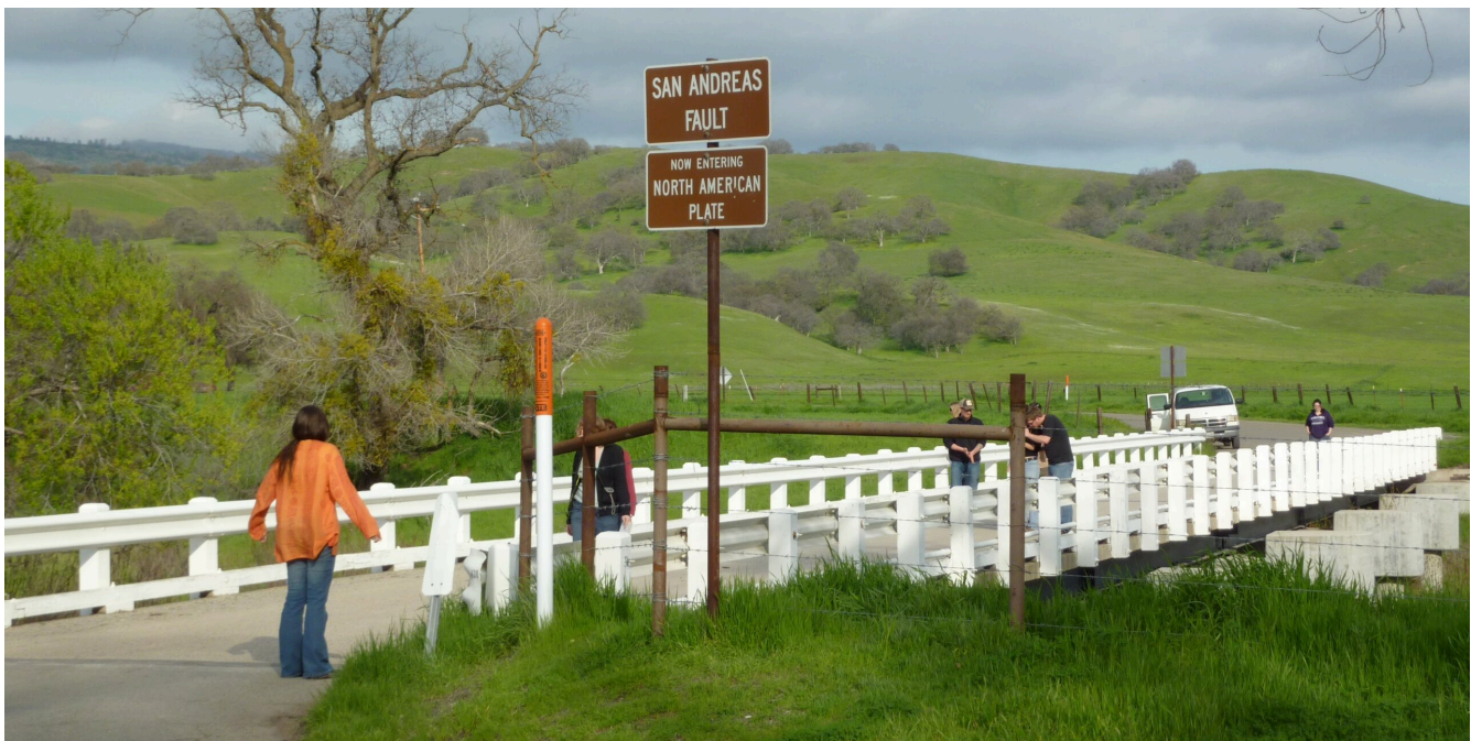
Figure 6.5.5 A bridge that spans the San Andreas Fault south of Parkfield California. The bridge deck is resting on concrete piers and it can slide as necessary when the foundations at either end move in different directions during an earthquake
