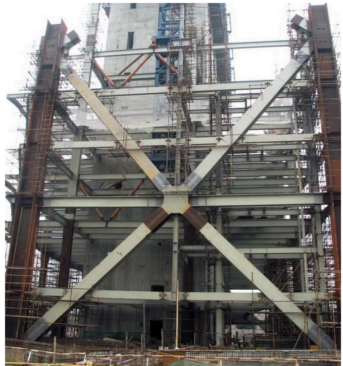
Figure 6.5.4 Strong Diagonal Bracing in the Pearl River Tower in Guanzhou, China
