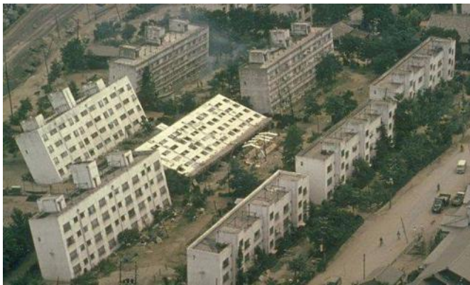
Figure 6.4.6 Collapsed Apartment Buildings in the Niigata Area, Japan. The material beneath the buildings was liquefied to varying degrees by the 1964 Niigata earthquake.
