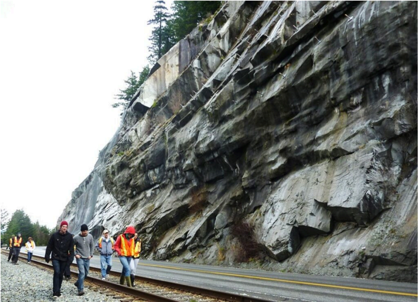
Figure 5.2.3 Site of the 2008 Rock Slide at Porteau Cove. Notice the prominent fracture set parallel to the surface of the slope. The slope has been stabilized with rock bolts (visible at the top) and holes have been drilled into the rock to improve drainage (one is visible in the lower right). Risk to passing vehicles from rock fall has been reduced by hanging mesh curtains (background).
