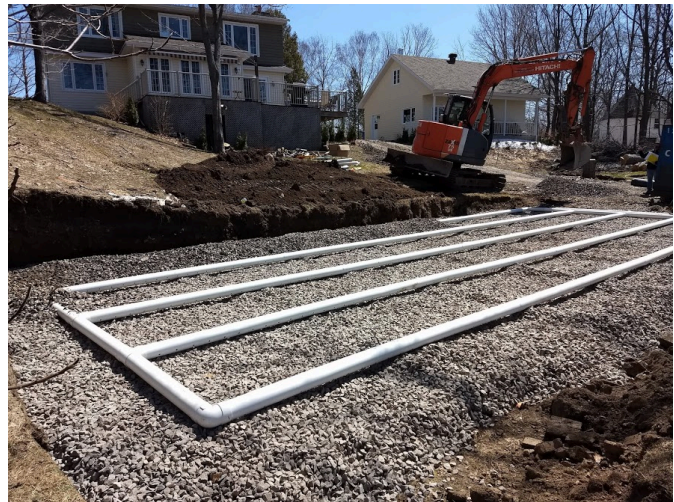
Figure 14.5.2 A Septic-System Drainage Field Under Construction. The perforated pipe will be covered with more gravel which will then be covered with soil.
