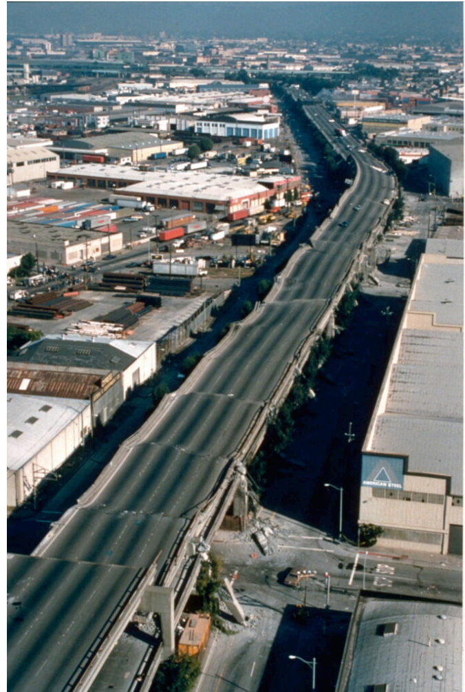
Figure 6.4.1 A Part of the Nimitz Freeway in Oakland California that Collapsed During the 1989 Loma Prieta Earthquake.
