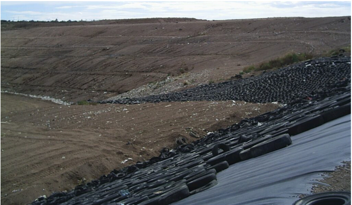
Figure 14.2.2 A Plastic Landfill Liner (Visible in the Lower Right). The rubber tires are waste and have been placed to protect the liner from damage from landfill materials and machinery.
