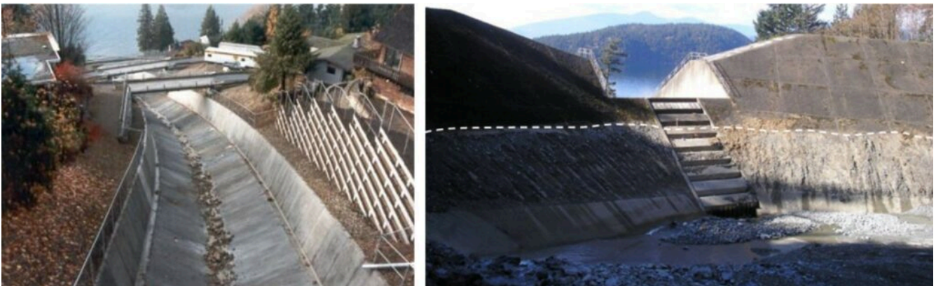
Figure 5.3.5 Two Strategies for Mitigating Debris Flows on the Sea-to-Sky Highway. Left: a concrete-lined channel on Alberta Creek allows debris to flow quickly through to the ocean. Right: a debris-flow catchment basin on Charles Creek. In 2010 a debris flow filled the basin to the level of the dotted white line.
