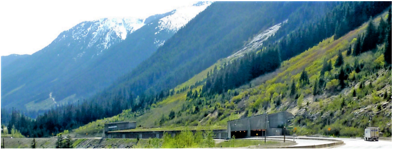
Figure 5.3.4 A Snow Avalanche Shelter on the Coquihalla Highway. The expected path of the avalanche is the steep un-treed slope above.
