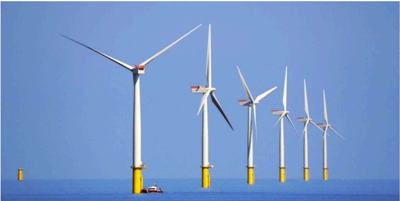
Figure 9.1.8 An Offshore Wind Farm Under Construction in the UK in 2011. These turbines are rated at 3.5 MW.
