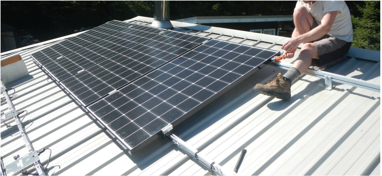
Figure 9.1.3 Installing Solar Modules on a Roof
