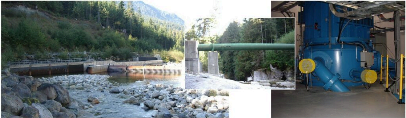
Figure 9.2.2 Components of a Run of River Hydro Project at Sechelt Creek, British Columbia. Left: the weir and head pond (at 360 m elevation); centre: part of the penstock; right: one of two 8 MW turbines at 10 m elevation.
