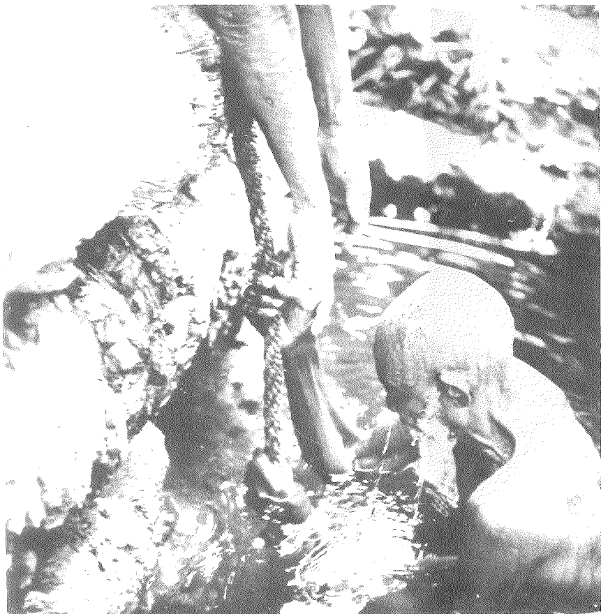
The "R'statts," well diggers since the tenth century in the R'hir wadi, Algeria. At the beginning of this century these men were still able to dig and maintain the wells, diving in the dark more than 80 m down to find the water, "this marvellous element which can bring life to all things" (the Koran). (Photo by Roger Viollet.)
