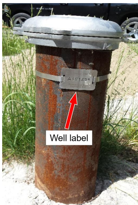
Figure 2 - Drilled well in Ontario, Canada, with well tag showing unique code (Well ID) affixed to the casing.
