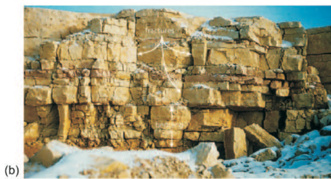
Figure 10.14 Field photographs of a quarry in the Carbonate Aquifer showing (a) bedding and well-developed karst features and (b) fracture sets.
