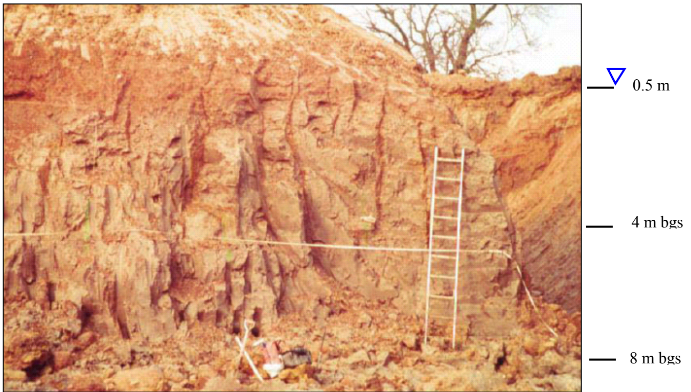
Figure 2.6 Photograph of fractures in a surficial clayey aquitard
