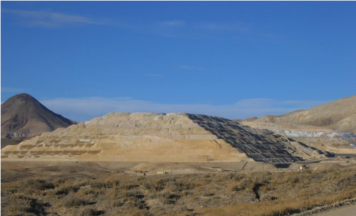
Figure 4 - A heap leach pile nearing the end of its operational life. The pile is approximately 100 m in height.
