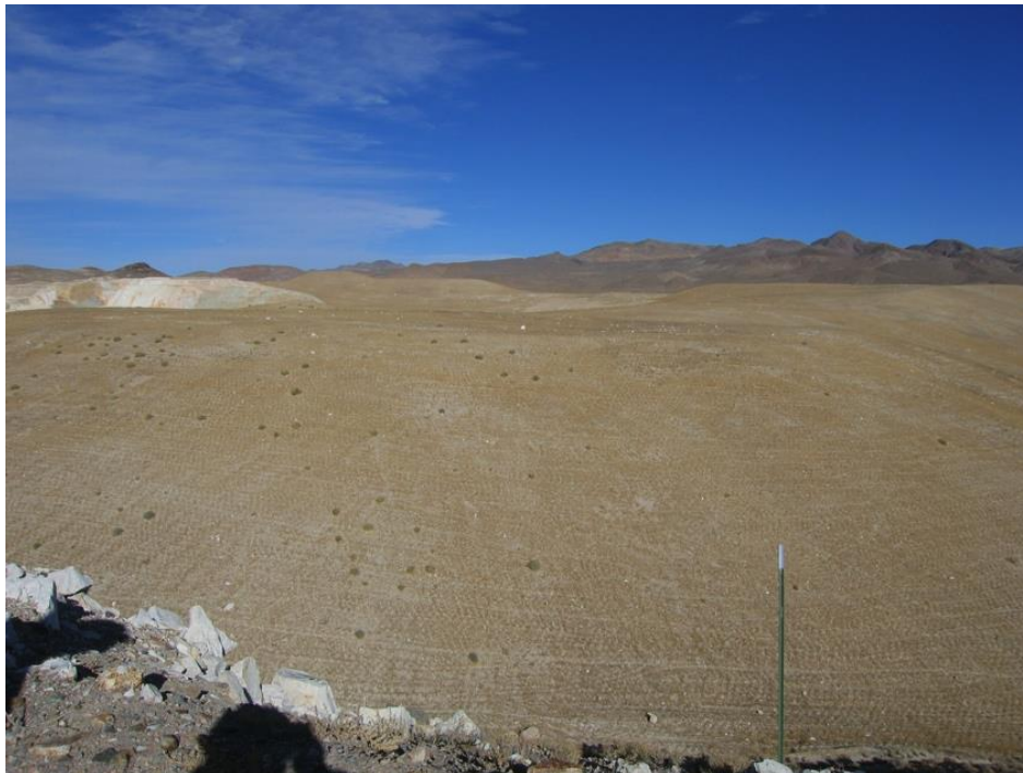
Figure 22 - Example of an isolation cover placed on a re-contoured waste rock pile.
