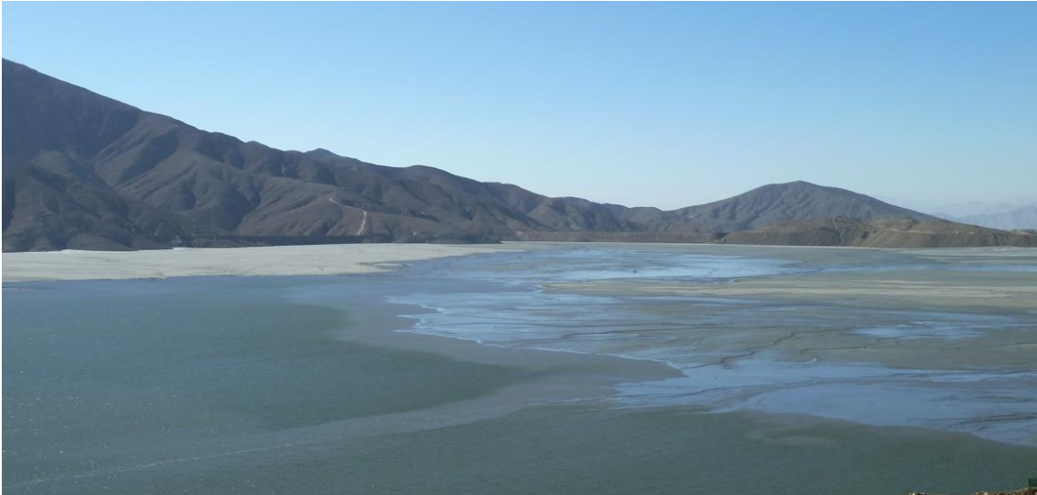
Figure 6 - Photograph showing the interior of a tailings storage facility with an older beach deposit where tailings release is not active (dry sandy area), a current beach deposit forming beyond the slurry discharge points located to the right, and the supernatant pond to the left in this tailings storage facility.
