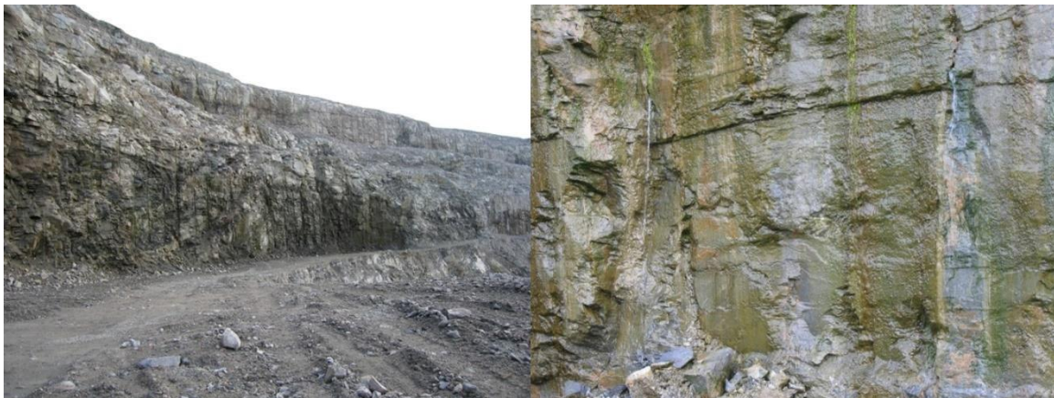
Figure 17 - Photo on left shows a seepage face near the base of an open pit, as indicated by general wetness of the rock surface. Photo on the right shows water emerging from discrete fractures farther along this same bench.
