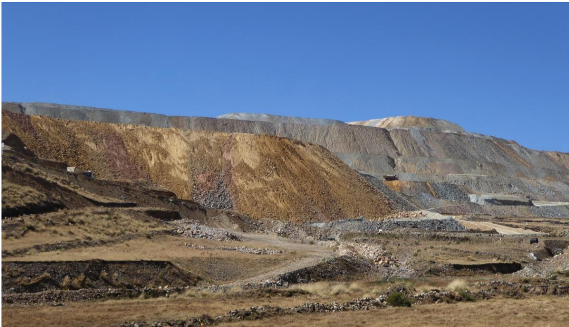
Figure 5 - Example of a multi-lift waste rock stockpile.
