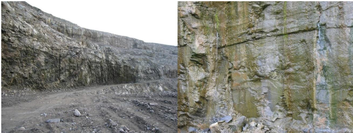
Figure 17 - Photo on left shows a seepage face near the base of an open pit, as indicated by general wetness of the rock surface. Photo on the right shows water emerging from discrete fractures farther along this same bench.
