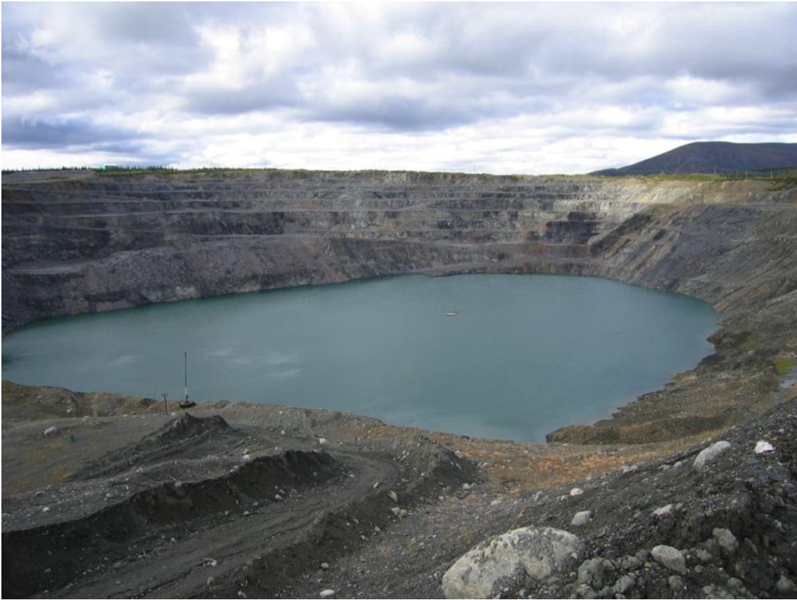
Figure 19 - Pit lake forming at a closed mine site. The pond level was rising at a rate of several meters per year, with the water level below the elevation of the subsurface spill point for the pit.
