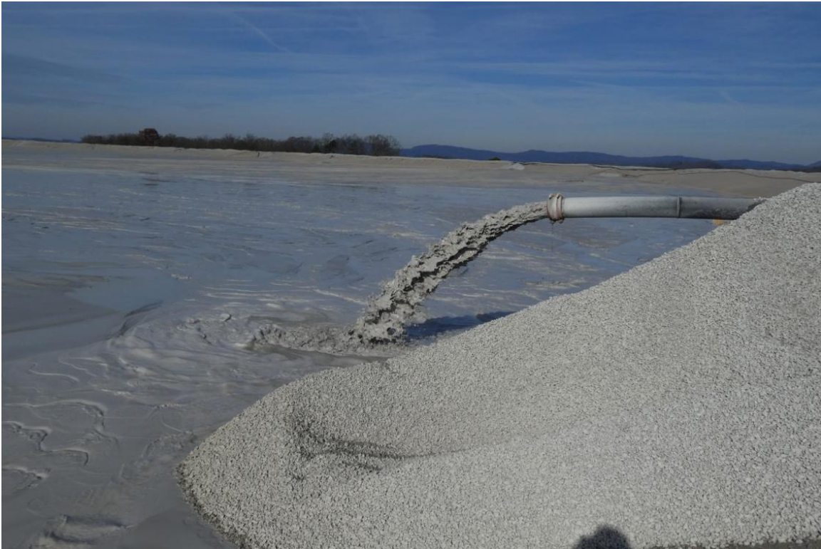
Figure 10 - Example of spigot discharge of tailings slurry from the embankment of a tailings storage facility.
