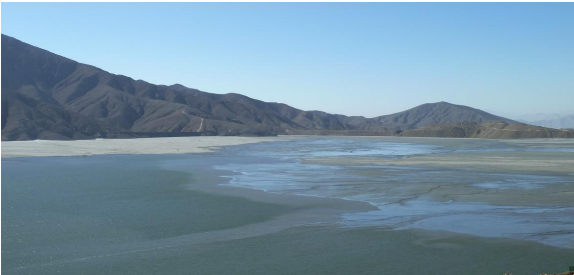
Figure 6 - Photograph showing the interior of a tailings storage facility with an older beach deposit where tailings release is not active (dry sandy area), a current beach deposit forming beyond the slurry discharge points located to the right, and the supernatant pond to the left in this tailings storage facility.
