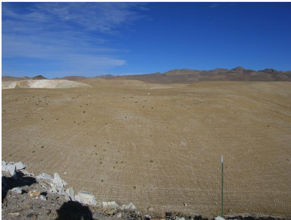
Figure 22 - Example of an isolation cover placed on a re-contoured waste rock pile.
